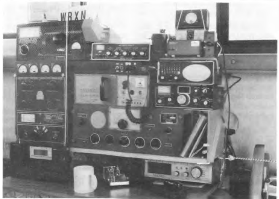
M/V SEA SPRAY/WRXN - Radio Equipment Console In Main Cabin
