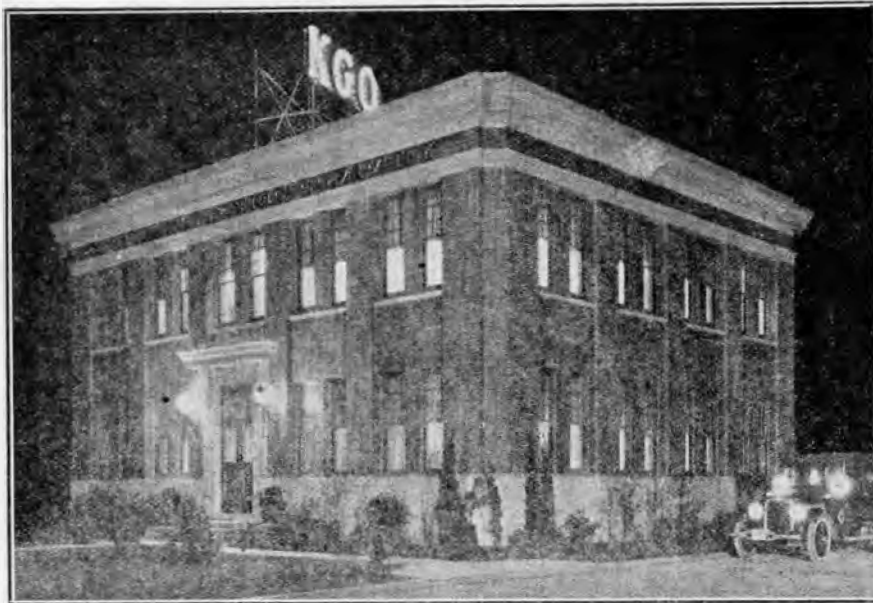
The General Electric Company's Broadcasting Station at Oakland, California.
